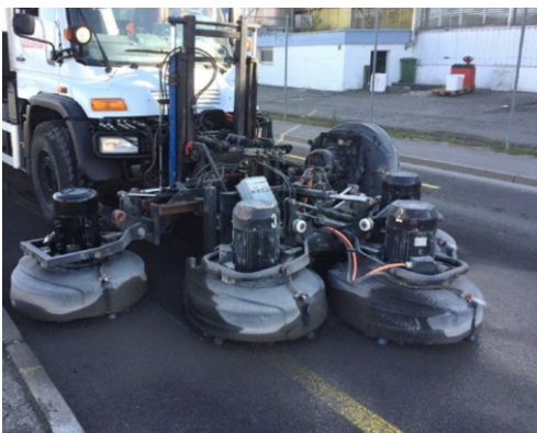
Figure 25: Milling of SDA coverings [Source: Hans Weibel AG]
