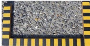
Figure 13: Comparison of washed concrete of different grain sizes with regard to acoustic pavement quality (Source: Grolimund + Partner AG)
